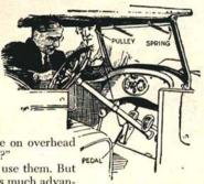
Drivers tired of swinging the wiper knob by hand found this homemade rig lightened a fatiguing job.
