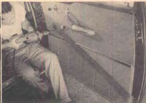
PLATED CLIP placed on door holds belt while not in use. Directions tell where to locate clip, but it's safer to probe with wire to be sure of hitting metal under fabric.
