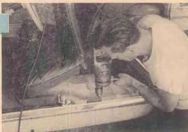
AIRCRAFT BELT can be used in small car or across one section of divided seat in larger one. You could adapt angle-iron anchor that writer used on Crosley to almost any car.
