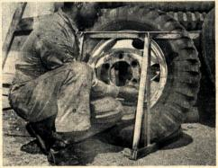
ADDING air to a big truck tire may seem perfectly safe, but accident records show otherwise. If lock rings are not properly set, the inrushing air may cause them to fly off with considerable force. Mechanics have suffered broken bones in this way. Some have been killed. For protection, Sgt. Isaac Guthrie, an Army motor mechanic, designed and built this shield. It's welded up from light angle steel, and can be slipped in place quickly.
