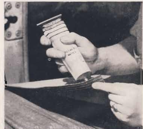
Worn floor mats can be repaired by applying patches of mat material with rubber cement used as adhesive
