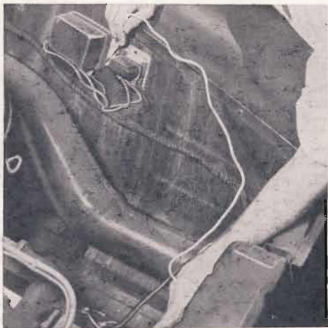
Regulator and generator frames connected together with copper wire determine poor ground condition
