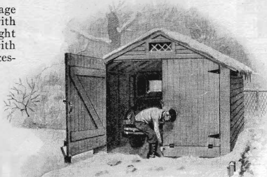
Fig. 1. A hinged section at the bottom of the door assures clearance in winter. Right: Diagram showing double hinge.
