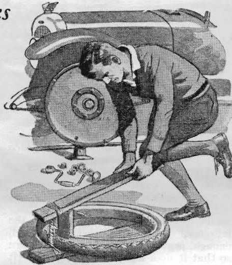
Fig. 1—Giant "nutcracker" is great help in mounting a stiff new tire on the clincher type of rim
