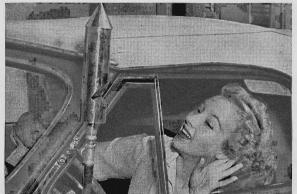
A SPEED-LIMITATION HORN for gas-and-rubber-saving drivers, toots its warning when the speedometer needle makes contact with a button set at the 35-mile mark on the dial. Contact opens a valve in the exhaust, which in turn blows the horn.
