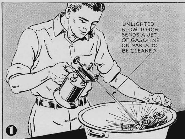
**1** **CLEANING DIRTY GEARS** and engine parts to which grease, sludge, and gummy deposits are clinging is simplified with a blow torch which has been filled with gasoline and pumped up to full pressure. Place the parts to be cleaned in a pan or a clean pail, and open the torch jet so that it shoots a stream over the dirty surfaces.—C.L.R.
