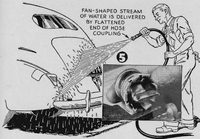
FAN-SHAPED STREAM OF WATER IS DELIVERED BY FLATTENED END OF HOSE COUPLING
