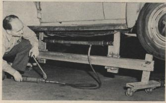
WITH two uprights braced against bent members of a car frame, the mechanic at left uses a small, portable pump to extend a hydraulic ram that will exert pressure to straighten them. The bent parts are then heated, and the Rogercraft Frame Press removed only after the metal has cooled. The press, made by the Hayward Implement and Engineering Co., Hayward, Calif., is eight feet long extended, and weighs 175 lb.
