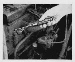
AN EFFICIENT, insulated tool for use on such jobs as testing car spark plugs, can be made from an old screw driver that has been discarded. Obtain a common rubber grip of the type used on bicycle handlebars, coat it on the inside with gasket shellac, and then fit it over the screw-driver handle. It may be found necessary to trim the handle a little in order to obtain a good fit.—F.H.
