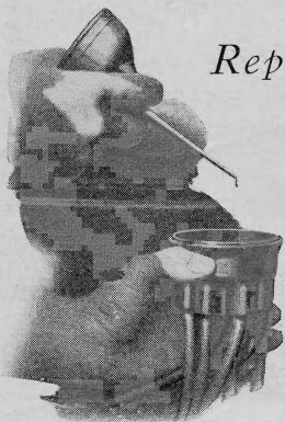
After scraping the crack, the cap is coated with oil
