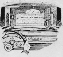
**Strips of reflecting tape** stuck on the edge of the garage-door opening, or on the door track if it protrudes, may prevent a scraped fender some dark night. Short strips placed at fender level are all you need to indicate clearances.
