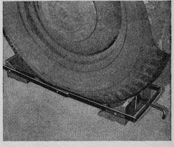
**Device Blocks Wheel.** An adjustable chock introduced by Modern Devices, Inc., Chicago, Ill., prevents a wheel from rolling in either direction. It consists of triangular wooden blocks held together by a metal frame, one block being removable so it can be set in place. A screw tightens the blocks. The frame folds for storage.
