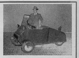
fore coming to the United States, this one had a single-beam frame, a radiator on each side of the 4-cylinder engine, and four speeds forward. It could attain a speed of 85 m.p.h. The streamlined front fenders were shaped to the wheels and moved with them when the car was steered.
