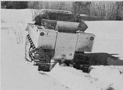
passenger cargo carrier sinks only 18" in light snow, and even under the worst conditions it beats struggling along afoot on skis or snowshoes. Capable of speeds up to 25 m.p.h., it overcomes most difficulties of terrain, ambling up a 45-deg. grade and over vertical obstructions as high as 19". Although designed for snow travel, it fords rivers less than 44" in depth on its own power and in deeper water becomes a boat.
