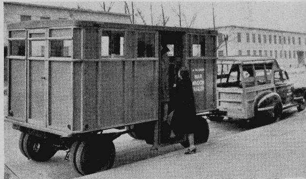
**LIGHT TIRES ON THIS TRAILER** and wood instead of steel construction save critical materials in the transportation of war-plant and other workers. The trailer mounts eight tires of the new Victory type that use but a few ounces of crude rubber compared to the 60 percent of crude required for heavy bus tires. The trailer seats 24 persons, and the converted sedan pulling it carries 15 more.
